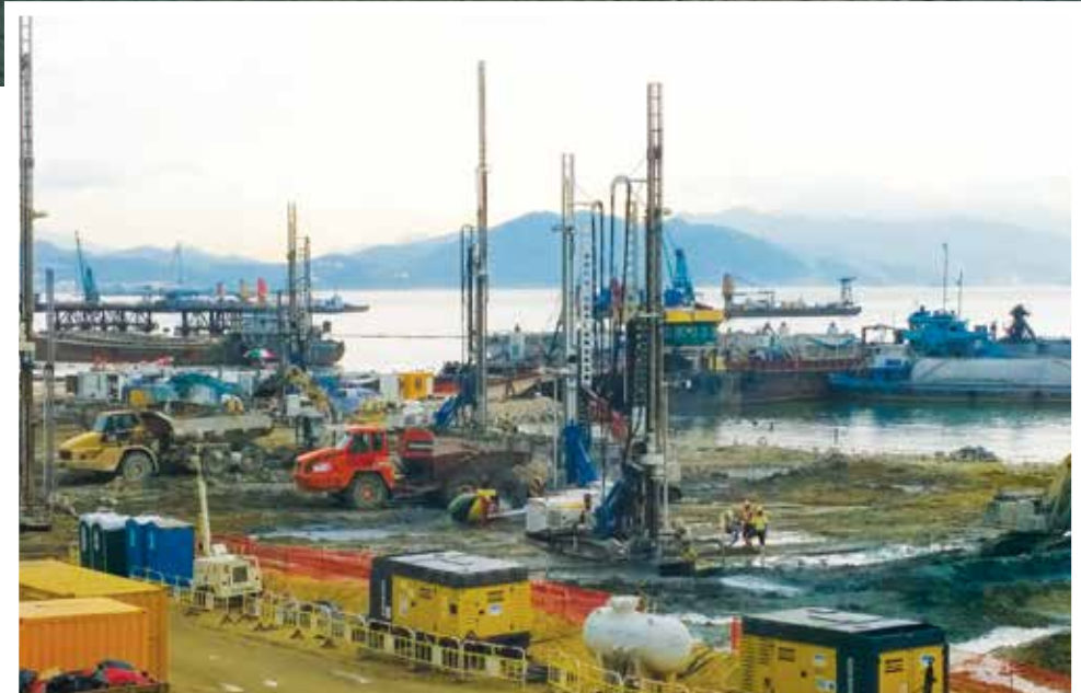
Right: Trevi Hong Kong complete the jet grouting construction in only two months, thanks in part to the reliability of their six Soilmec drilling rigs.
