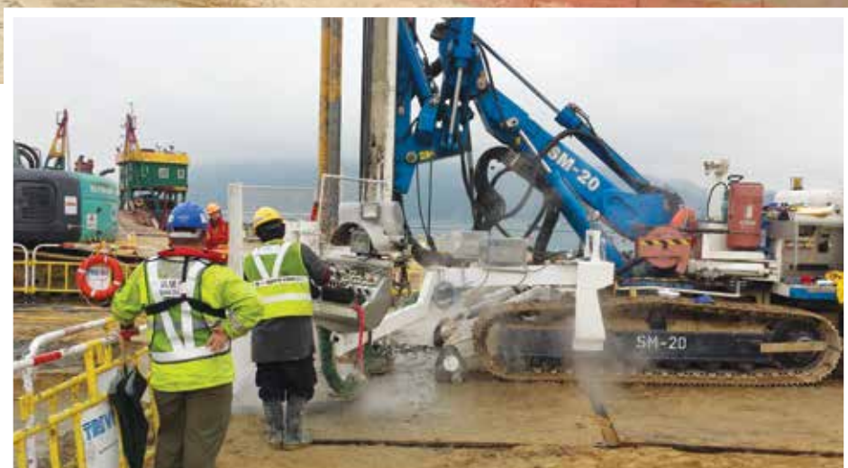
Trevi Hong Kong depended on Soilmec drilling rigs to install 450 jet grout columns, helping to stabilize an artificial island at the centre of the Hong Kong-Zhuhai-Macao Bridge project.
