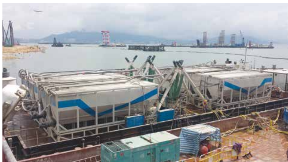
Parked alongside the island, two barges were equipped with 14 silos and four grout mixing plants to keep up with the high consumption rate of cement grout – 1,200 cubic metres per day.
