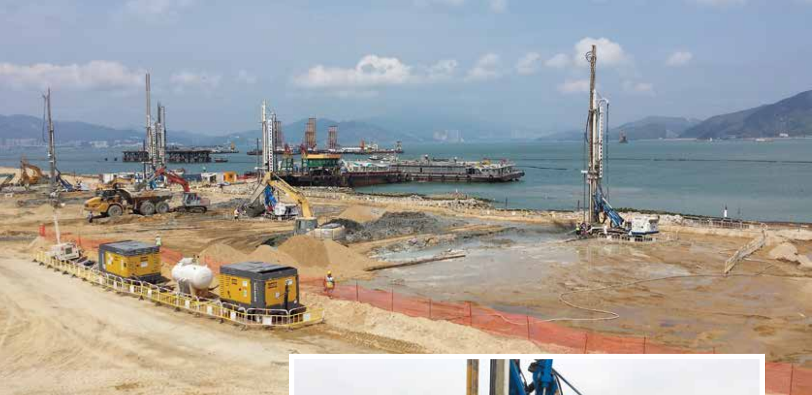
Soilmec PSM-20 rigs jet grouting on an artificial island just northeast of Hong Kong International Airport.
