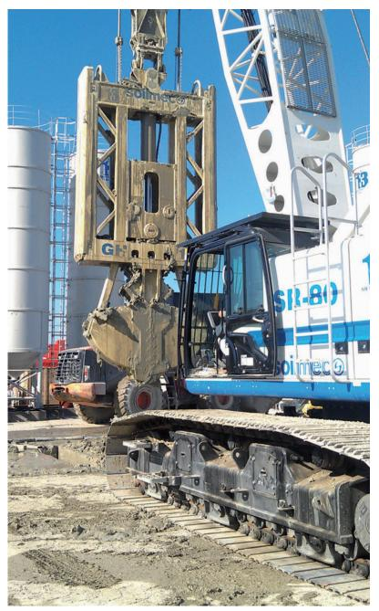
Diaphragm wall construction requires that a proper sequence of works is followed. A rectangular-section tool is generally used to remove the soil, thus creating a rectangular excavation.
