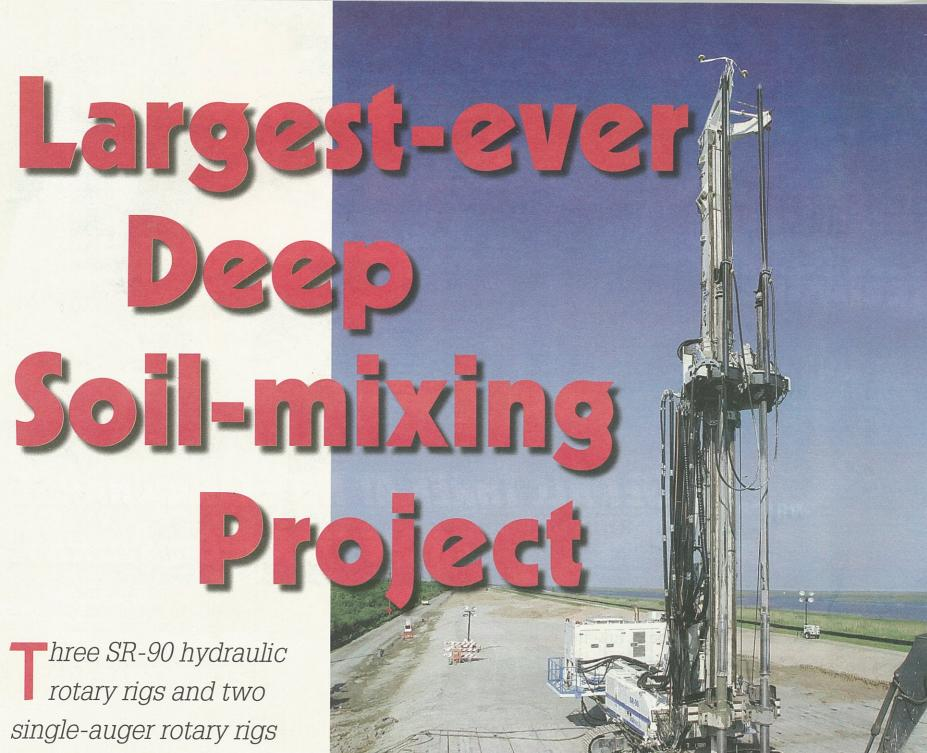
Three SR-90 hydraulic rotary rigs and two single-auger rotary rigs (SR70 and SR80) are at work in New Orleans on the biggest deep soilmixing job ever performed in the United States.
