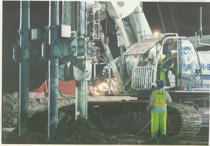
The machines also ensure the correct positioning of the columns, thanks to the Drilling Mate System, which provides full monitoring of all vital
