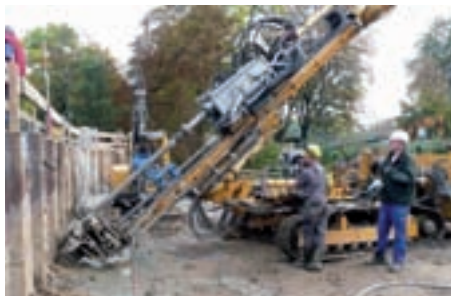
SonicSampDrill's MidSonic rig anchor-drilling in Speyer Rhineland, Germany
