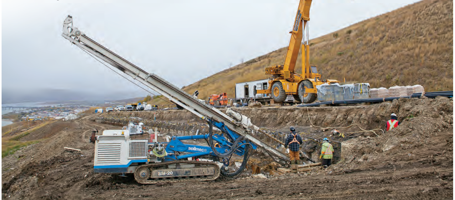
Soilmec SM-20 rig installing ground anchors on a sloping hillside (Courtesy of Doublestar Drilling)
