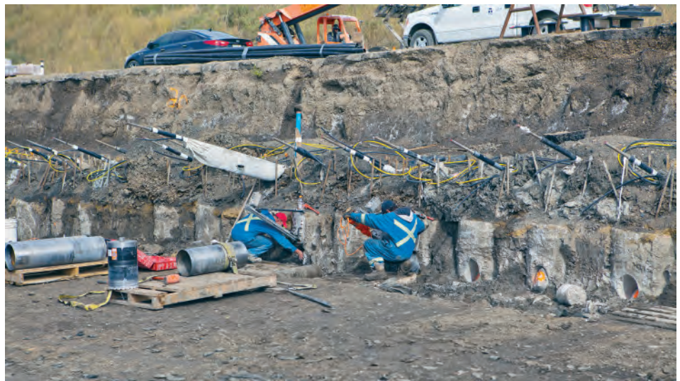
Two rows of tiebacks installed at 25 and 30 degrees to horizontal (courtesy of Doublestar Drilling)
