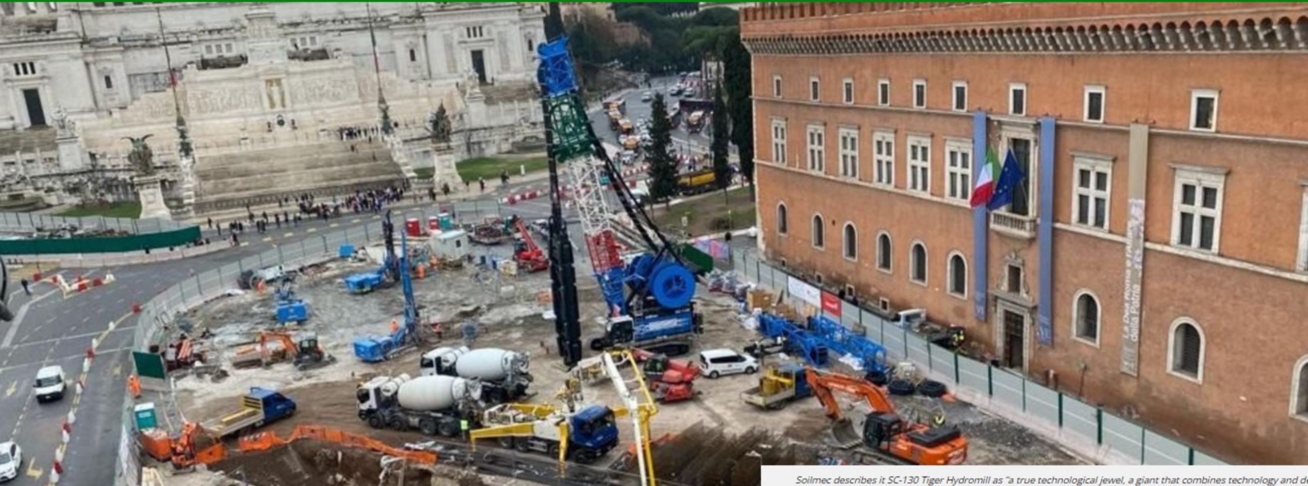
Soilmec describes its SC-130 Tiger Hydromill as “a true technological jewel, a giant that combines technology and design to speed up work times and operate with greater precision and in smaller spaces, reducing noise and vibrations on the surface. The machine is imposing but also compact at the same time.”
