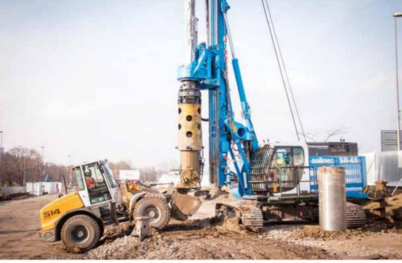
tomer can choose either the spin-off Soilmec system (it leverages the cinematic energy generated by the high-rotation speed, up to 135 rpm, and is unparalleled when using the auger) or the new click-click system, which is very efficient using the bucket and especially in very cohesive soils.
