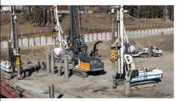
As part of that work, Ki installed temporary H-piles and lagging, a type of earth retention system, on the east and west side of the parking facility to allow for excavation and protect adjacent structures like sidewalks and roads.
